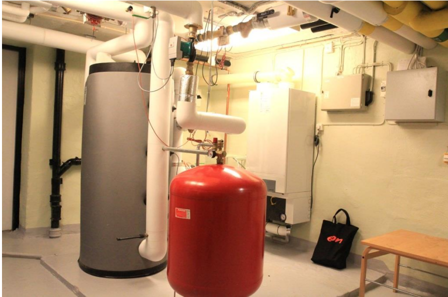
Figure 6 Boiler room after installation of new gas boiler and heat storage
