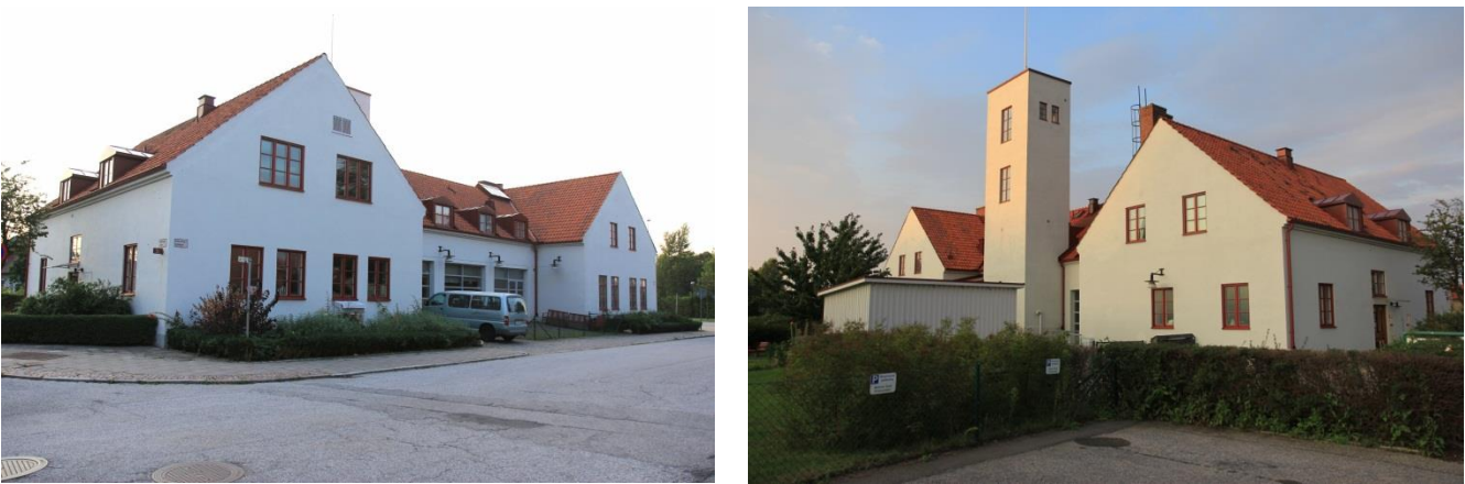
Figure 1. Limhamn old fire station now used for day care activities
