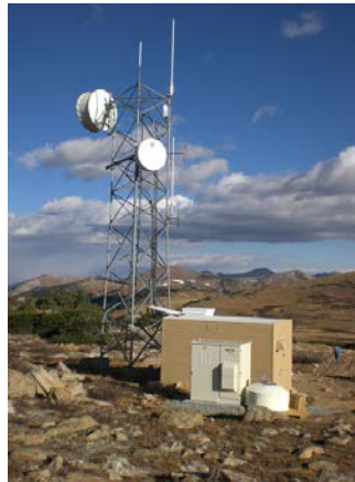
Ballard ElectraGen™-ME methanol fuel cell backup power system installed at a telecom base station site
