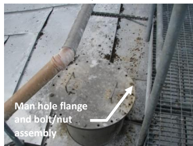
Figure 3 Overview of detected leakages (arrows indicate precise location of the leakages)
