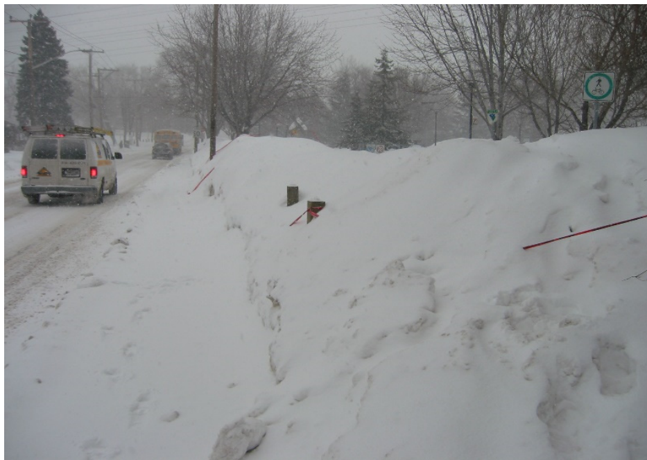
17.5 Snow dyke made to prevent the river water to flood the road; the snow was transported and compacted with a snow blower; February 2 nd , 2014
