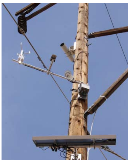
Figur 22 Installerat Span Sentry system [24]
