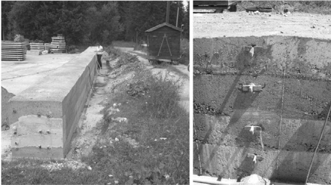
Figure 69 - Photos of the RCC block with the strain sensing cable embedded within it (Moser et al).
