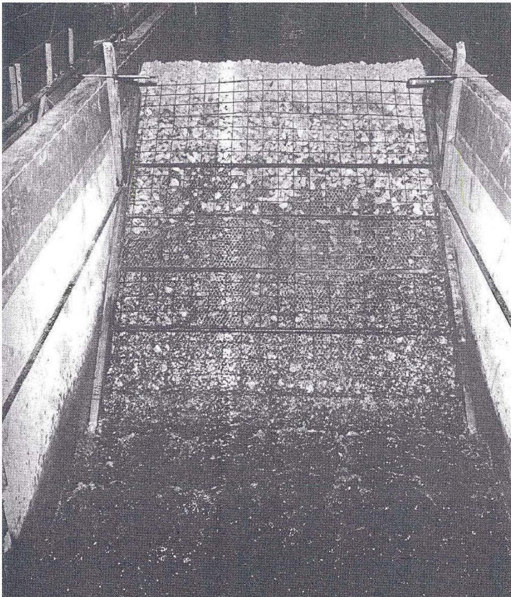
Figure A.2 The dam used in the experiments as seen from downstream.
