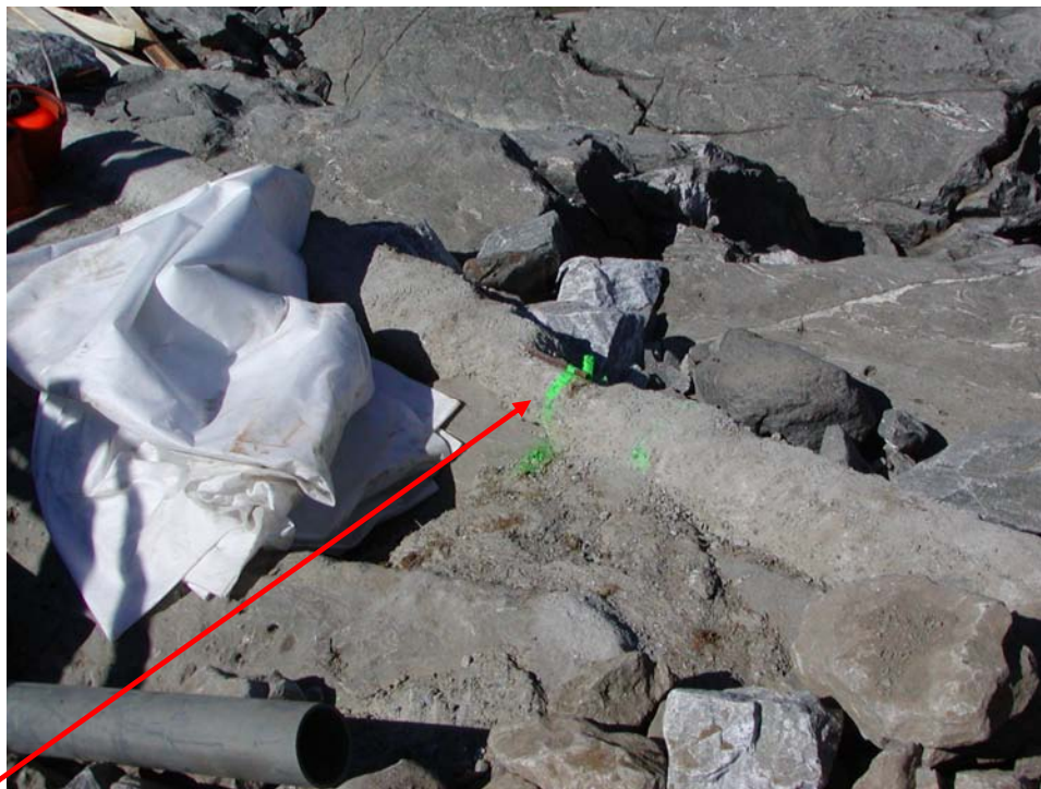
Figure 25 The “centerline” for the embankment marked at the concrete sill downstream of the embankment.
