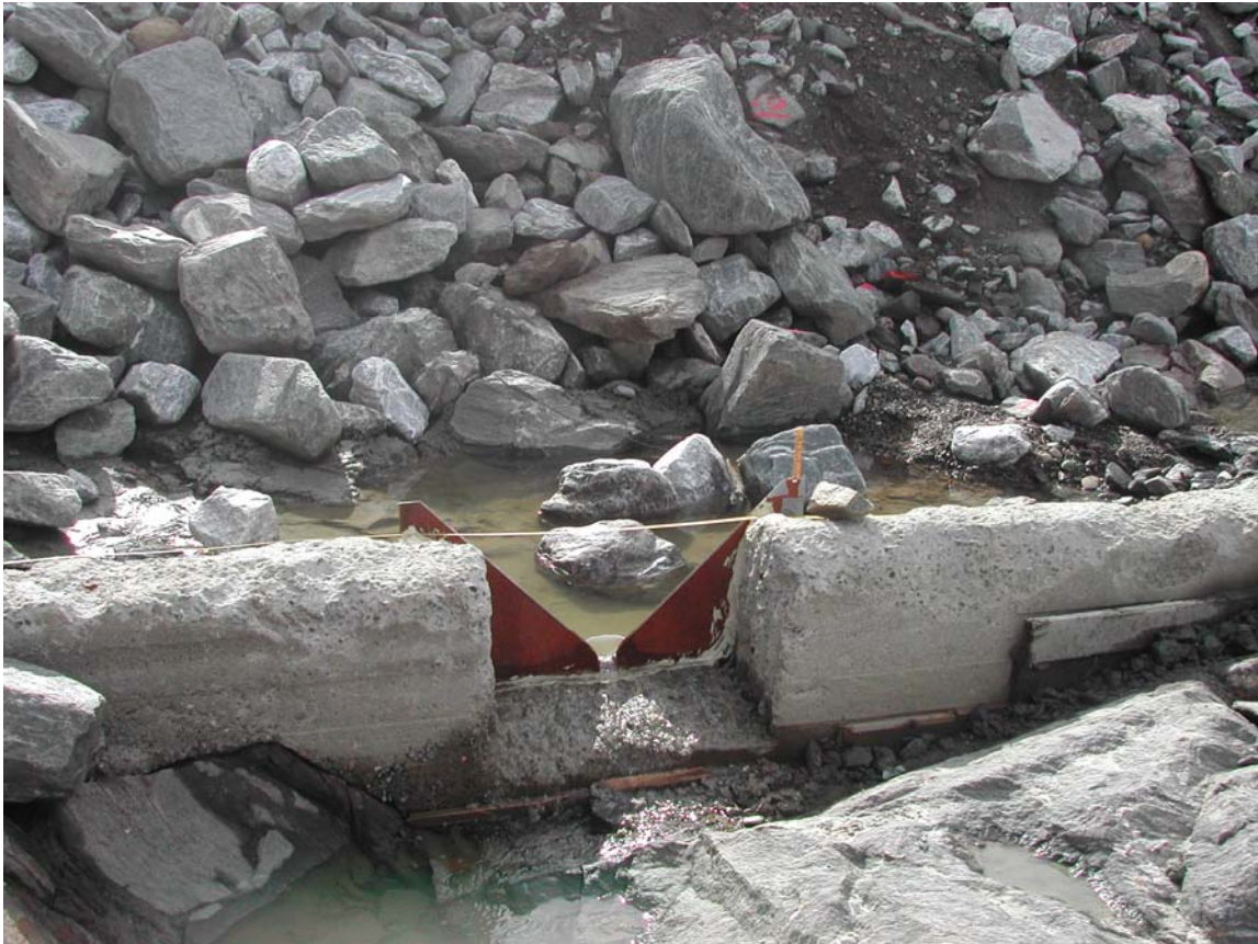
Figure 7-2 Seepage flow weir downstream the dam.
