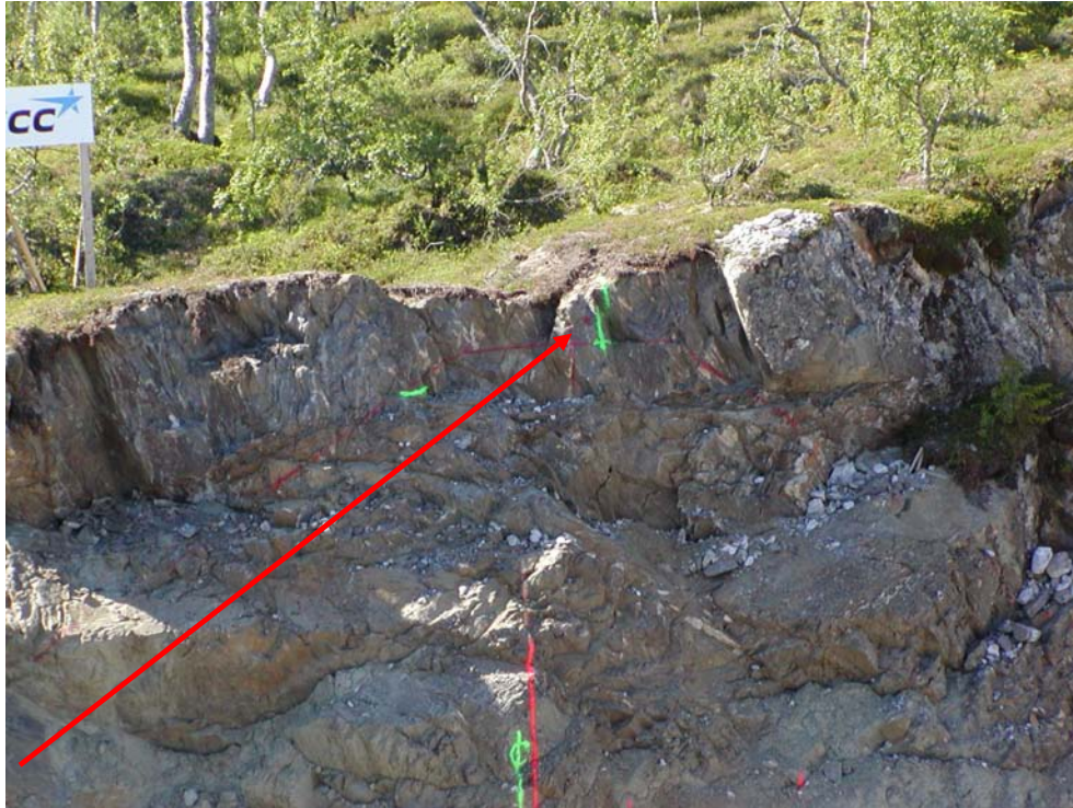
Figure 24 The zero point at the left abutment
