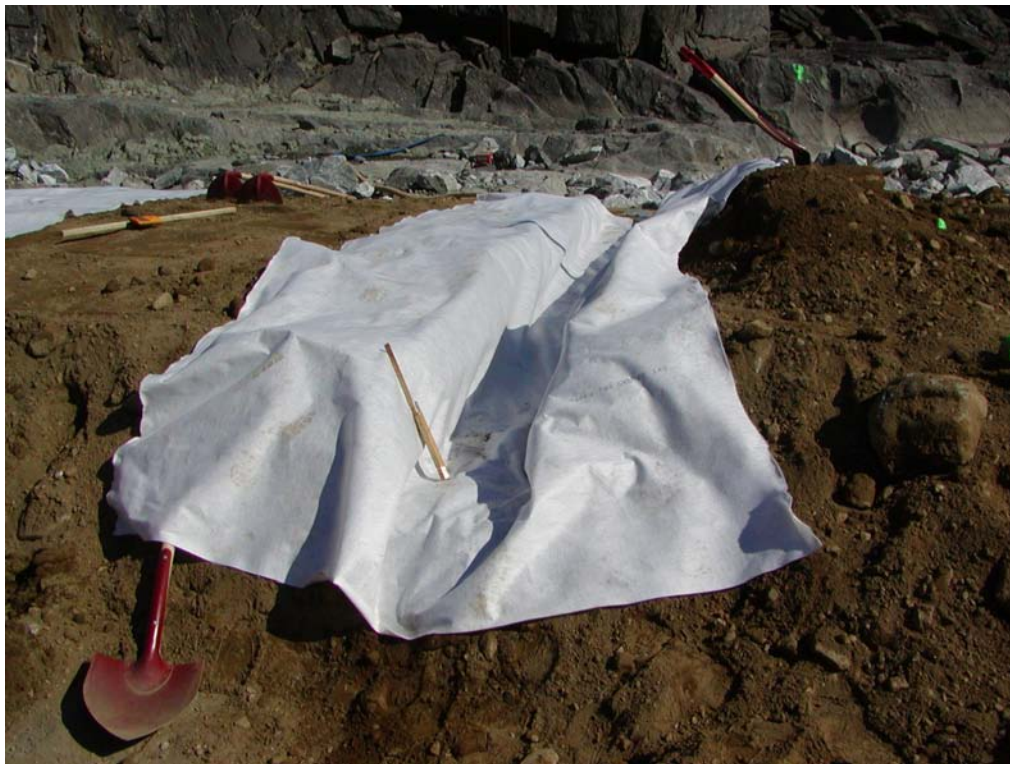
Figure 19 Defect A, filter fabric is arranged before the placing the gravel into the excavation
