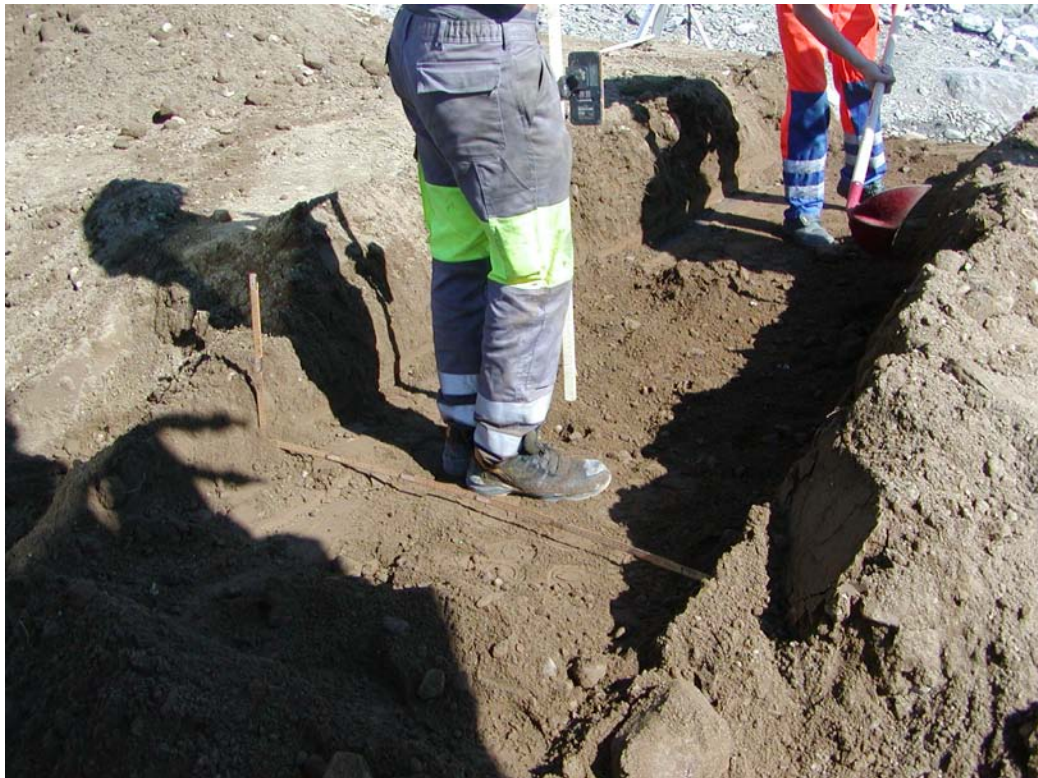
Figure 21 Defect B, excavation
