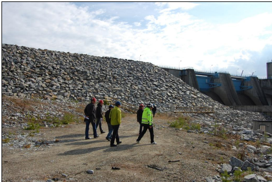
Figure II.3 Site visit to Hällby dam (May, 2011)
