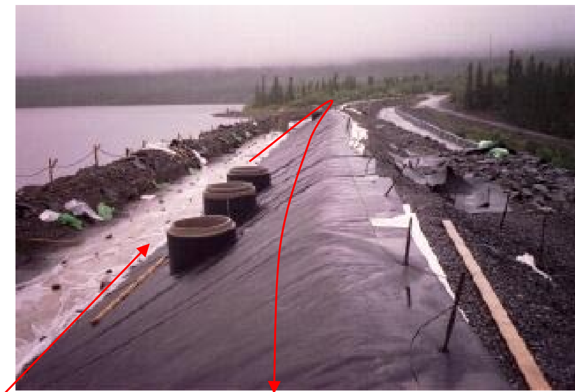
Figure 10 Location of the cables on the membrane. (The picture was taken during construction of the dam).
