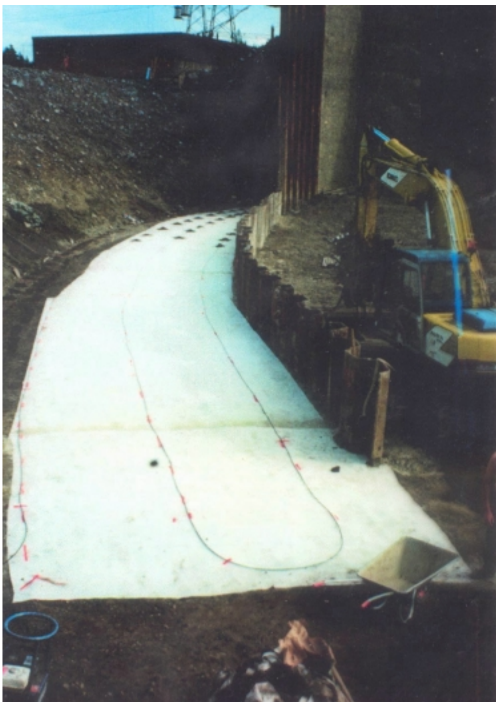
Figure 4 Geomembrane connected to the sheet pile at El +274.0. Two fibre-optic cable loops can also be seen on the top of the geomembrane and on the downstream filter. (Photography by Graningverken AB)
