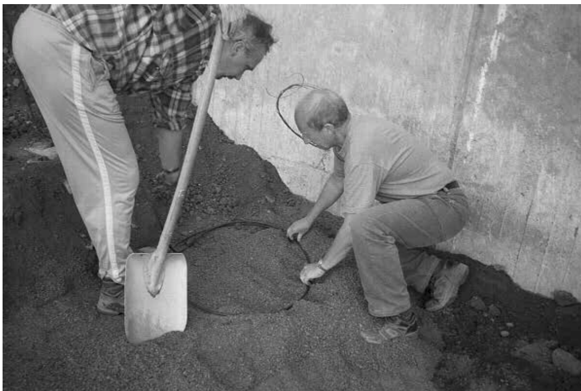
Figure 7 Installation of the upstream fibre, with an extra loop close to the vertical rise along the concrete wall.
