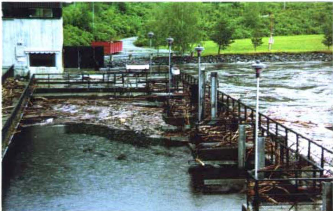
Figure 3.14. Floating debris of a smaller size during a high flood.
