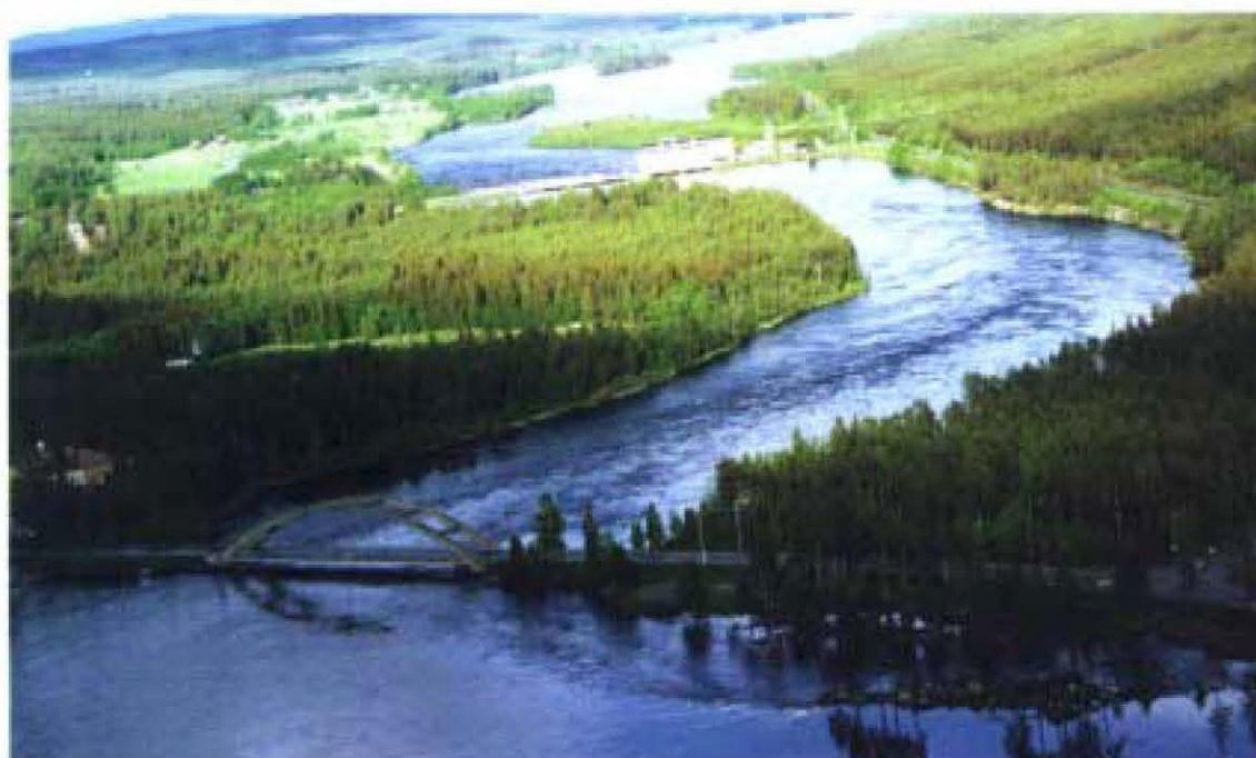
Figure 3.1. The photograph shows head losses upstream from Stugun Power Plant in high flow conditions. The losses are experienced at both the bridge and further upstream (lower part of picture).
