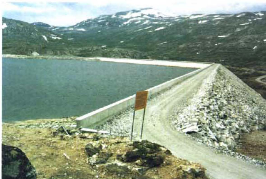
Figure 4.6. Wave protection (parapet) to avoid overtopping of the dam crest.
