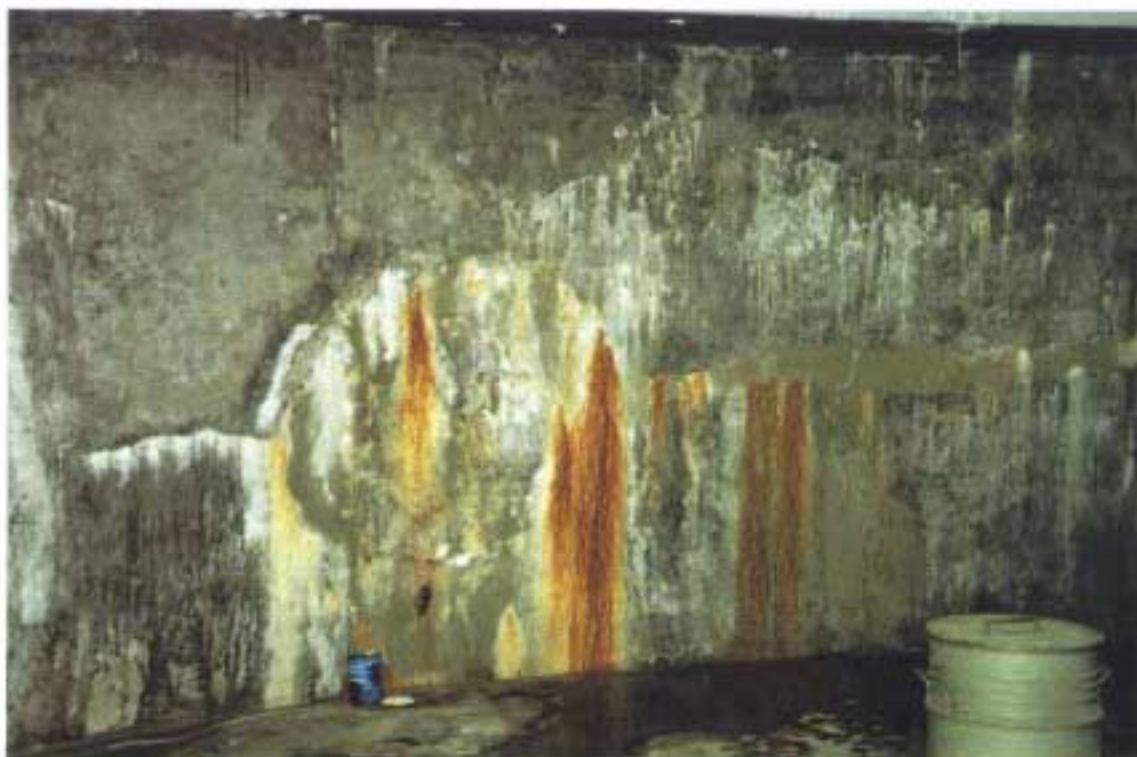
Figure 8.1. Layers of lime on wall.
