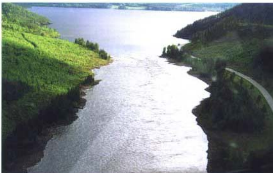
Figure 3.4. The photograph shows head losses under high flow conditions at the outlet of Gesunden. During normal flow, it is the same water level as far as Krångede Power Plant 1 km downstream.
