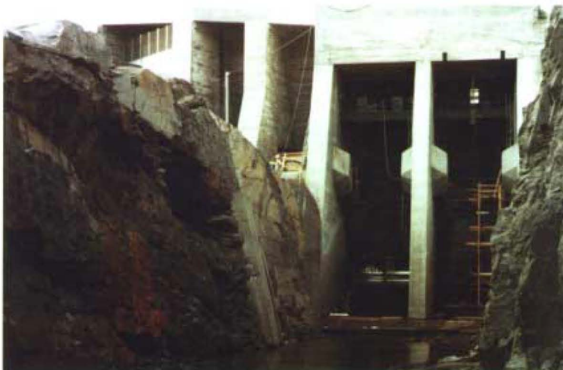
Figur 6.7. Spillway where the rock was damaged during a test.
