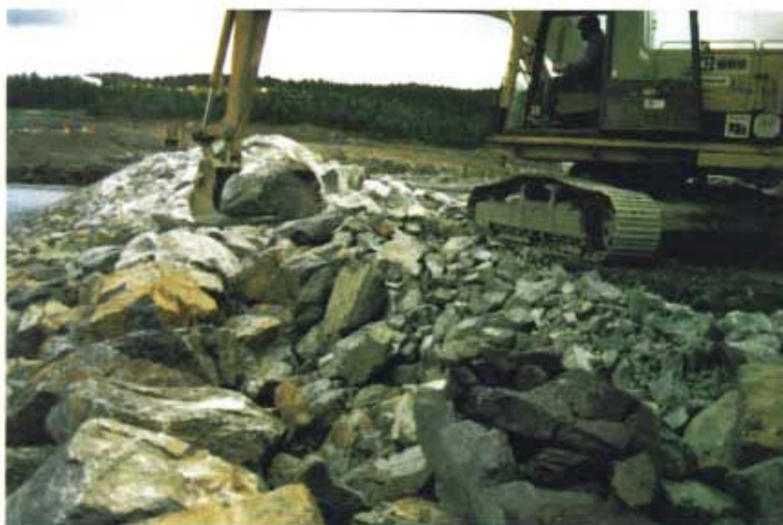
Figure 4.3. Laying boulders with an excavator for the upstream erosion protection at a rock-fill dam.
