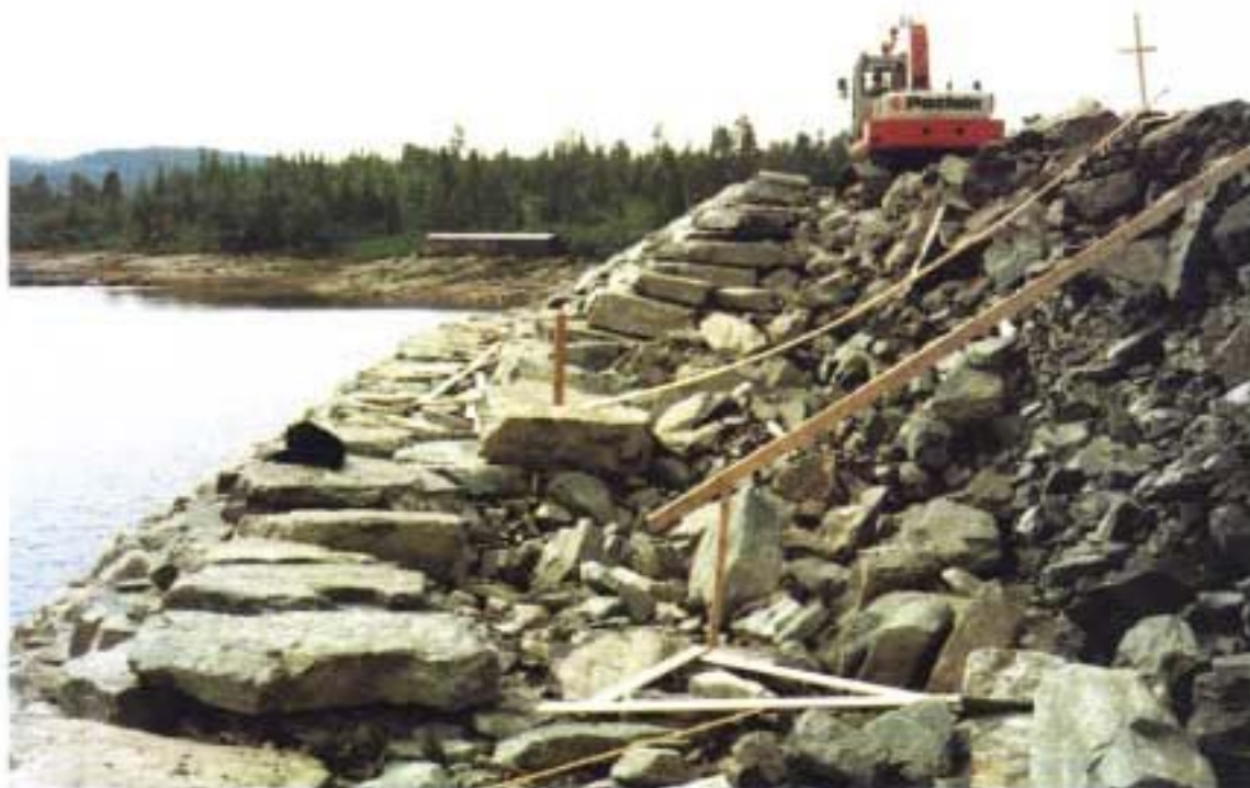
Figure 4.4. Provision of erosion protection with a surface layer of carefully arranged narrow and flat-sided boulders.
