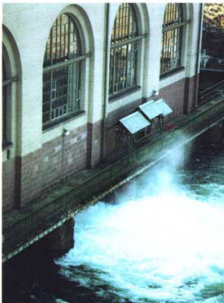
Figure 6.4. Spillway test at Motala Power Plant (no damage).
