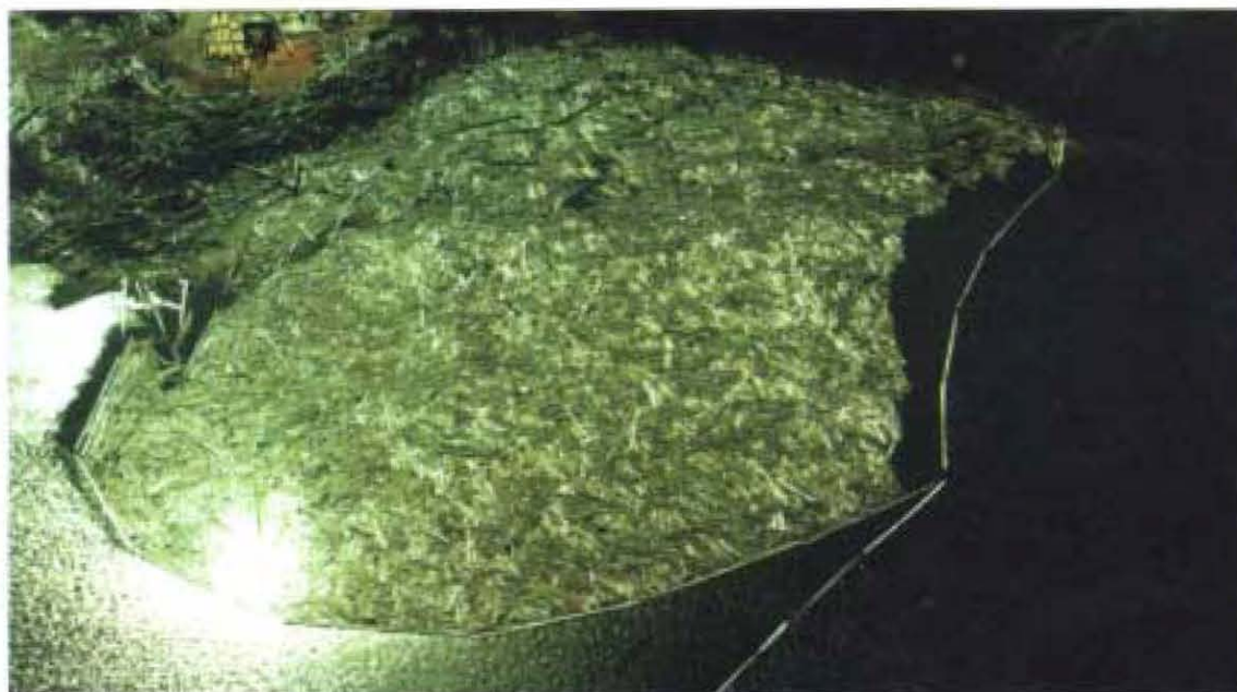
Figure 3.13. Collecting or retaining floating debris with the aid of log booms in Canada.
