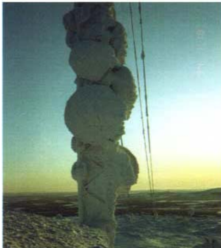
Figure 3.8. The equipment must withstand the sometimes hard climatic conditions in the northern Scandinavia. The photo shows a communication link tower.
