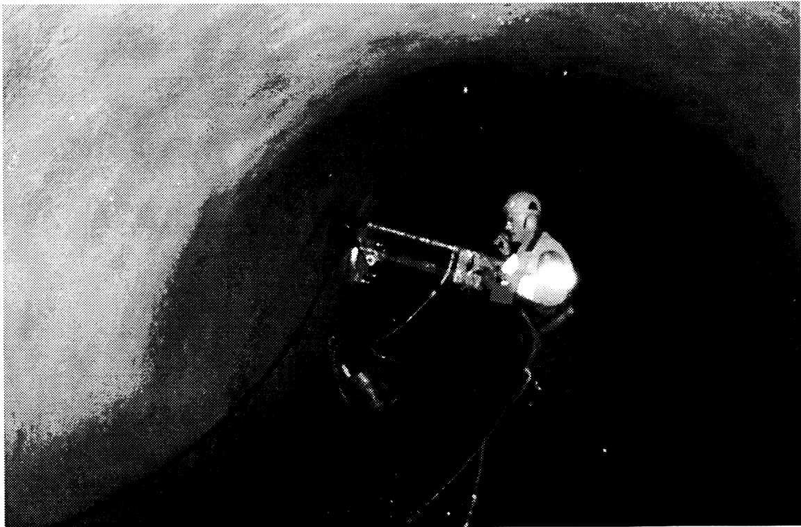
Figur 4.25 Kärnbörning i vägtrumma, Lerum Core drilling in "tube bridge", Lerum
