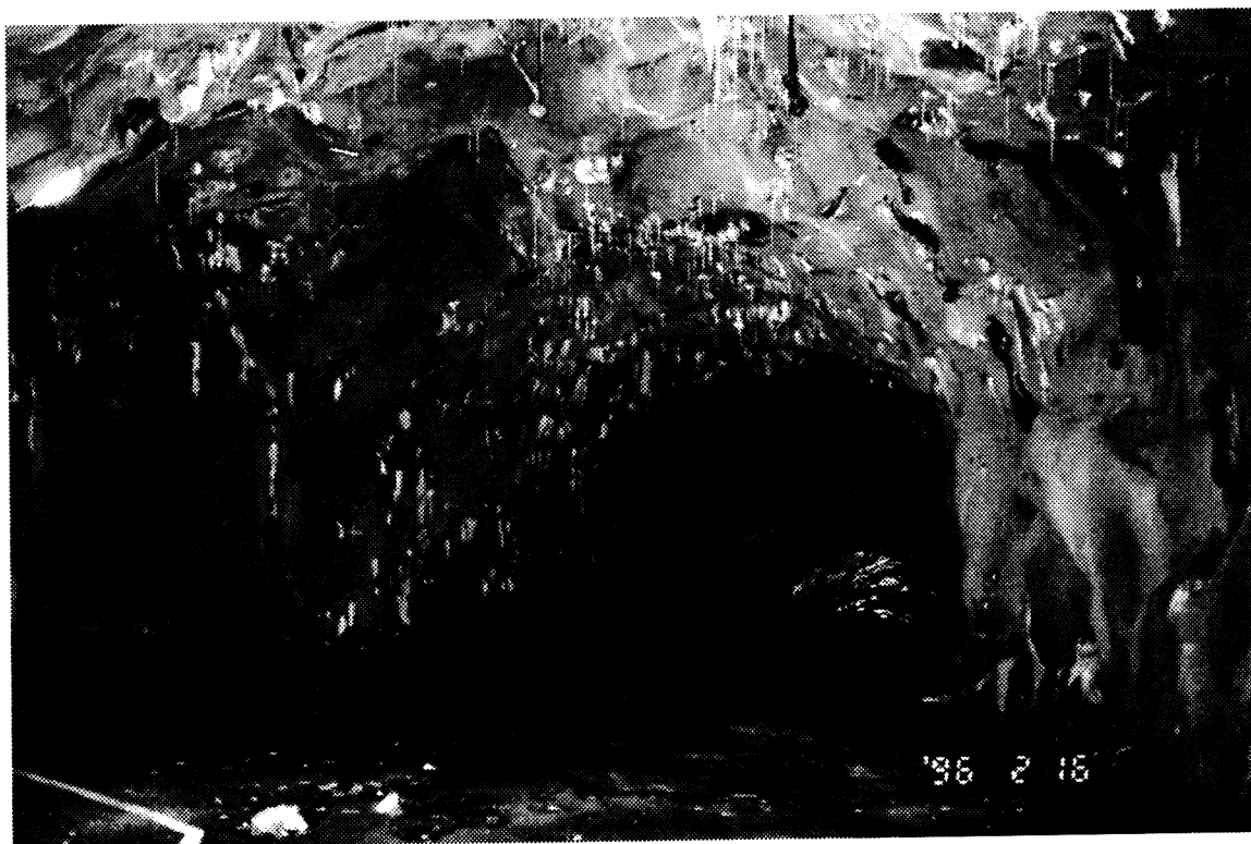
Figur 4.8 Kalkutfällningar i ventilationsort, Umluspens kraftstation. Lime deposits in ventilation gallery, Umluspen power plant.
