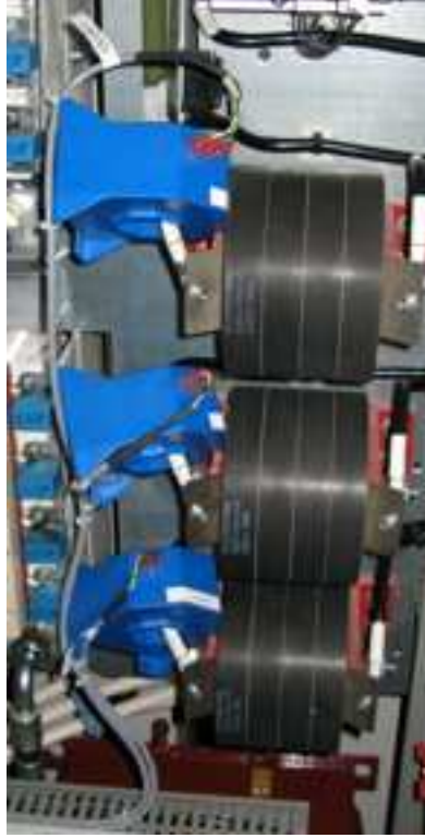
Figure 5.4: DC crowbar resistor with a current sensor (blue).
