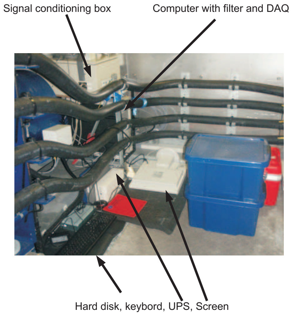
Figure 7.6: Physical arrangement of the signal conditioning box and data acquisition computer, at the rear of the nacelle.
