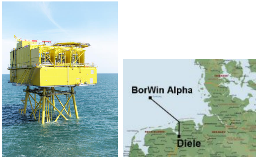
Figure 9.1: BorWin 1 offshore HVDC hub
