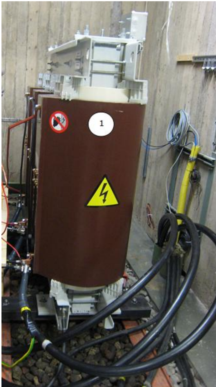
Figure 6 Dry type transformer used in laboratory test (during preparation): (1) Transformer
