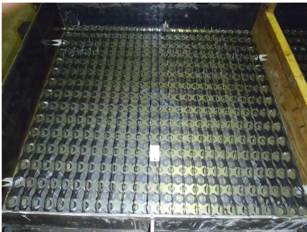
Figure 10 Photo prior casting of slab SC1 with cell reinforcement
