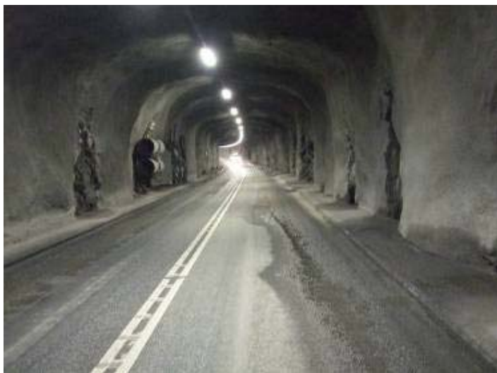
Figur 1 Muskötunneln (The Muskö tunnel).
