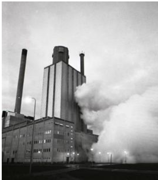
Fig. 5. Simulated steam explosion at Marviken. The steam coming out of the reactor building fell later down as a luke-warm rain. Photo by Ingvar Anehed [NT2011].
