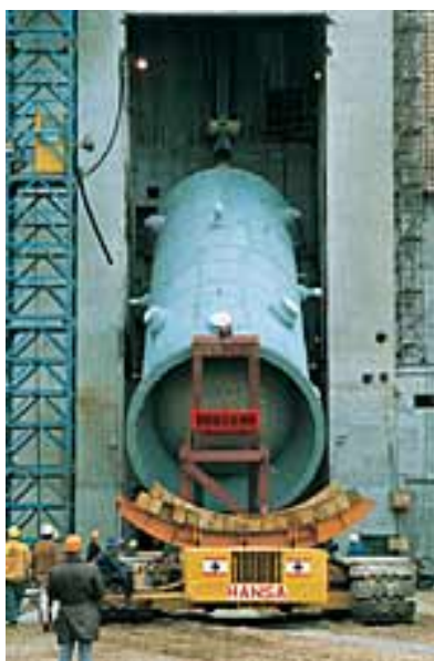
Fig. 3. RPV during plant construction (Courtesy BKAB).
