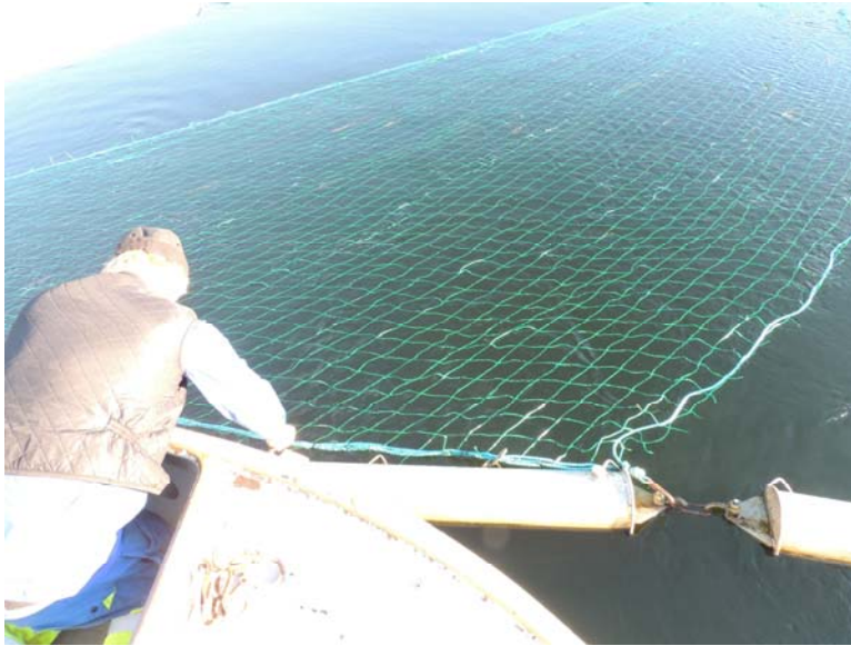
Figure 5. Ice booms with mounts for nets.
