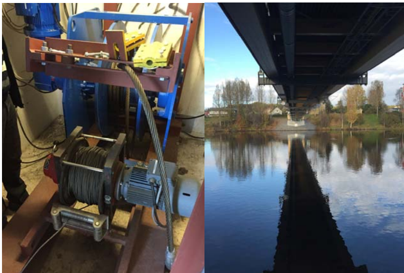
Figure 6. To the left, machinery for winding of the cable for mounting of the net. To the right, the location under a bridge where the ice nets were mounted.
