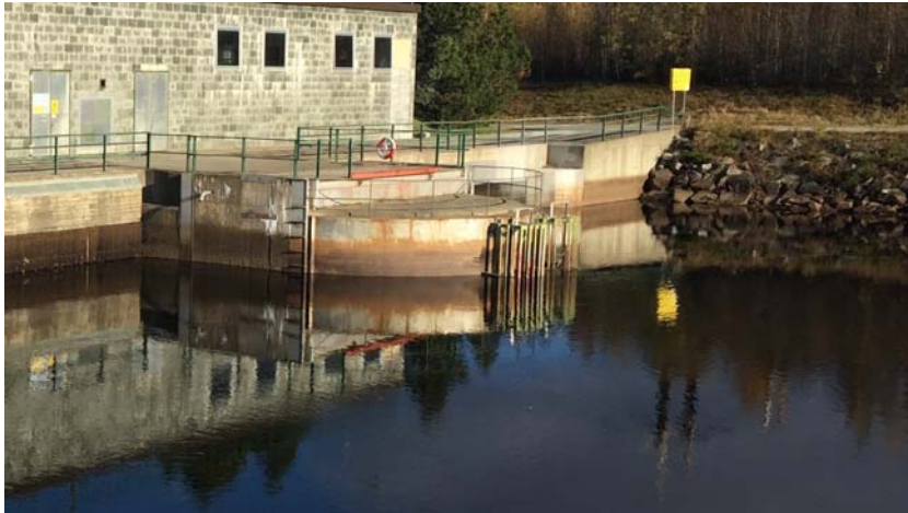
Figure 7. The water intake gates at Kvistfossen.
