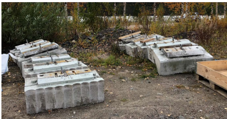
Figur 31 - Demonterade statorfundamentplattor.
