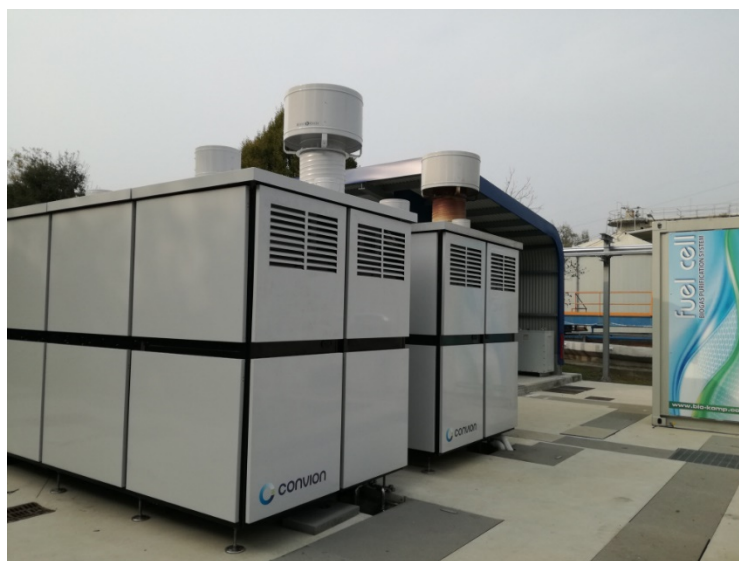
Convion FC system. Courtesy of DEMOSOFC.
