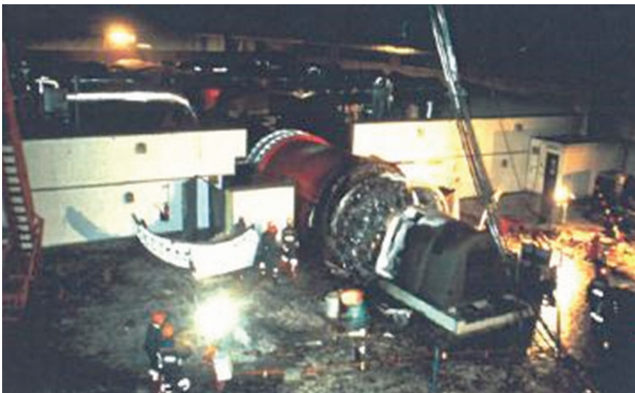
Figure 5. Explosion of retaining ring caused by stress corrosion cracking (Barsebäck)
