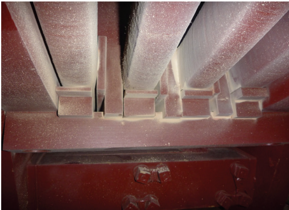
Figure 54. Fretting in round connection
