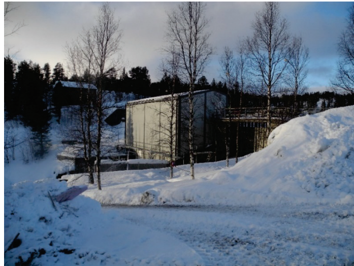
Figure 5-25 Floodgate rebuilt with a climate wall.
