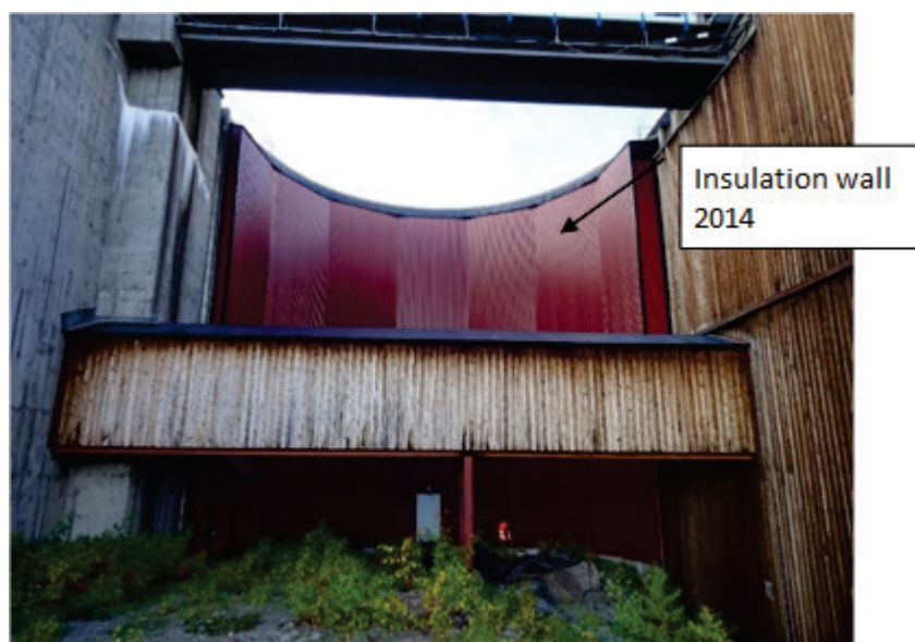
Figure 5-15 The arch (Westberg-Wilde, 2014).
