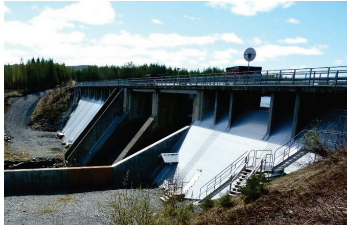
Figure 5-50 The dam in 2017 with a new heat-insulating climate wall
