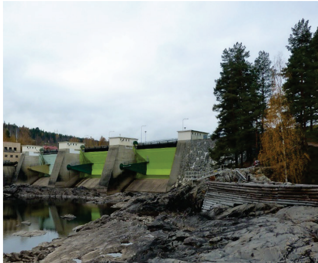
Figure 5-3 Downstream side of the spillway dam.
