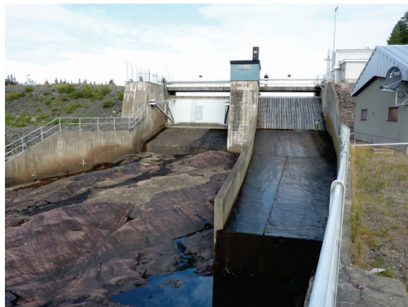
Figure 5-8 Downstream side of the spillway dam. P1=studied middle pier.
