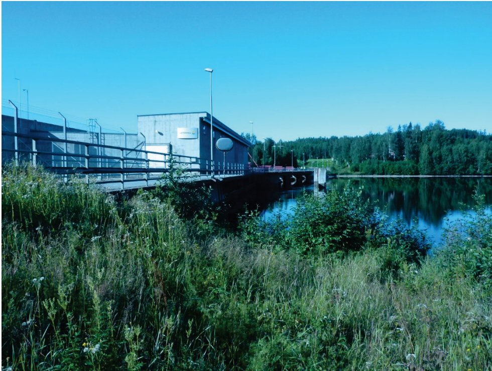
Figure 5-11 Upstream side of the power house
