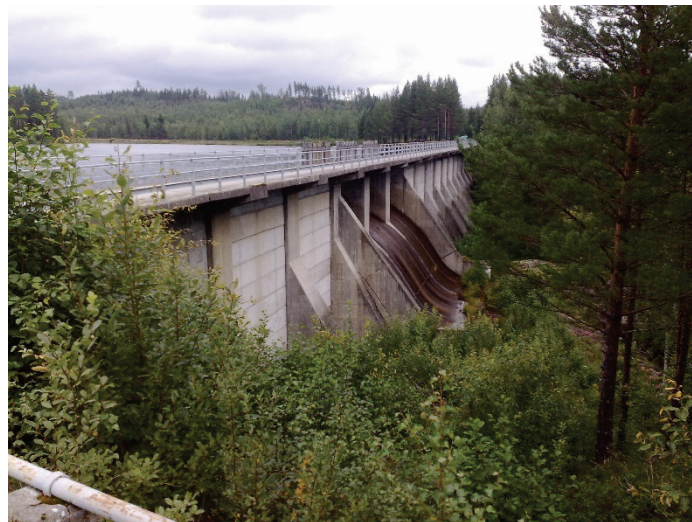
Figure 5-27 The concrete dam in dam unit 1.
