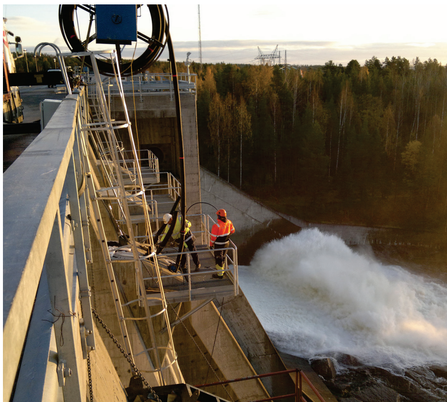
Figure 4-18 Ongoing installation of pre-stressed cable in buttress dam.
