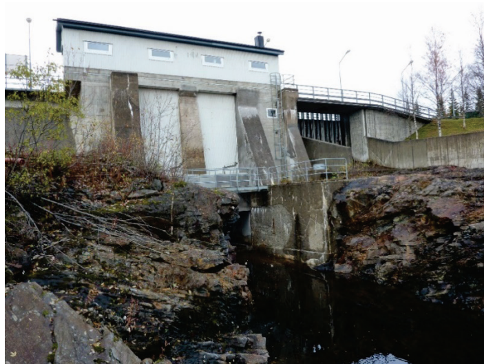
Figure 5-23 The regulating dam
