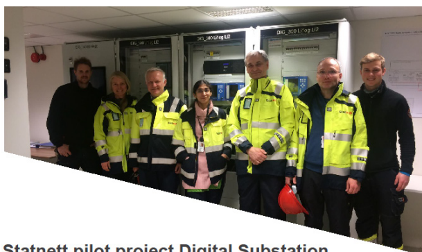
Statnett pilot project Digital Substation with IEC 61850 process bus
