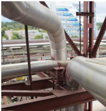
Figure 55. Piping at PAO Acron Chemical production facility.
