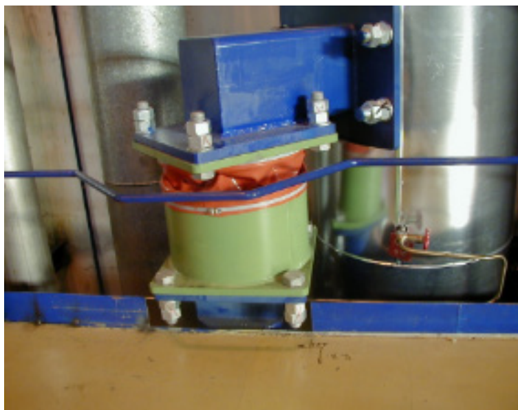
Figure 47. VD damper at the RA11 in turbine hall. Damper's piston attached to the piping, housing to the TH gallery floor.
