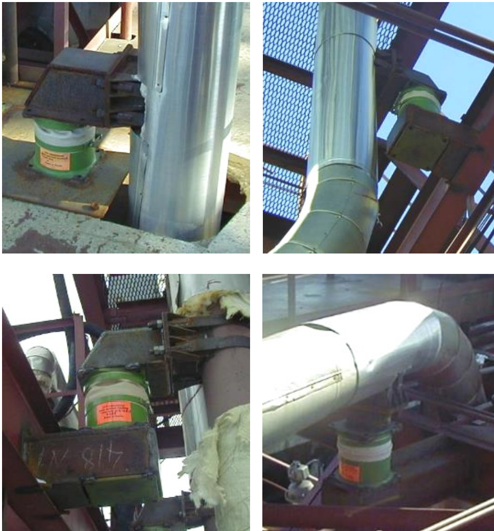
Figure 57. Dampers installed on the piping of waste heat boiler.
