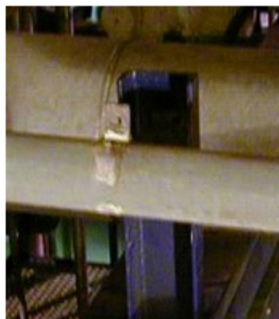
b) fatigue collapse of elastic support.
