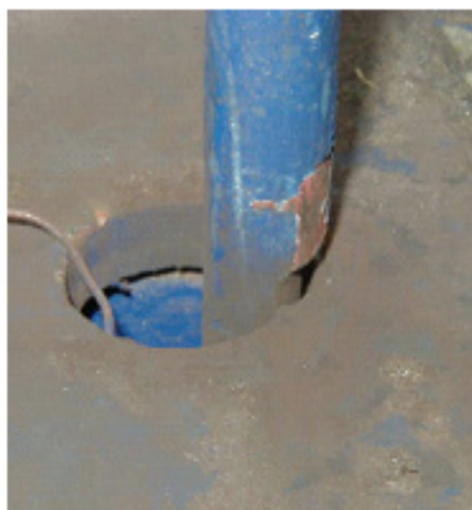
a) wear of the rod hanger.
