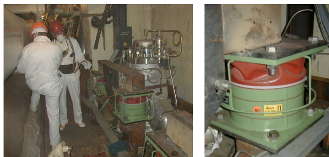
Figure 65. Vibration protection of the MSL safety valves at Chernobyl NPP, unit 3.
