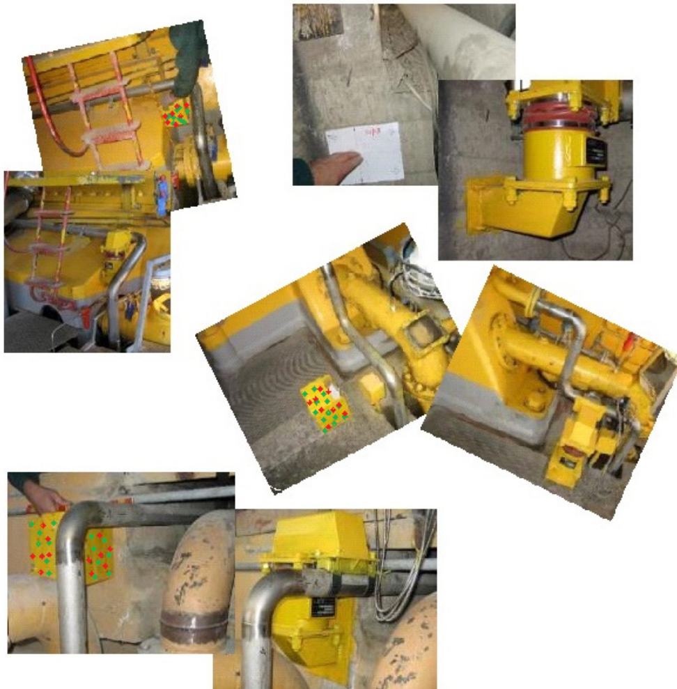
Figure 52. Places for dampers installation before and after dampers installation. The speckled yellow box is a mockup of damper.
