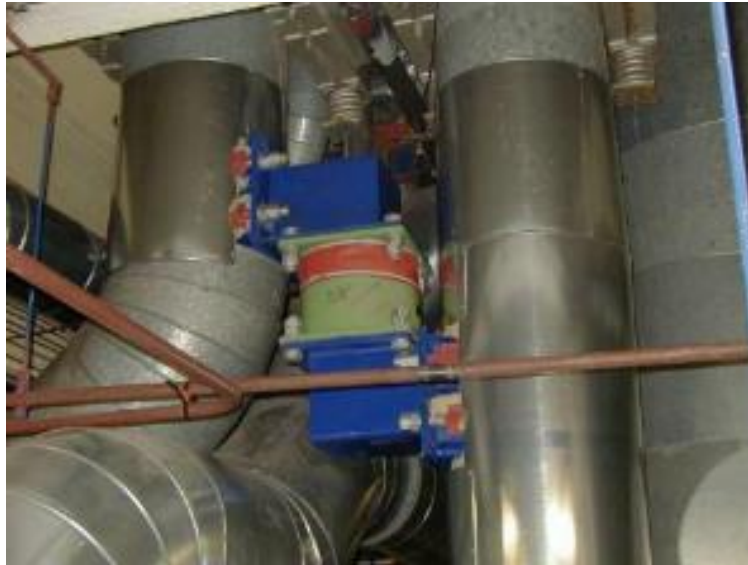
Figure 48. Connection of two RA piping with different dynamic properties by VD damper
