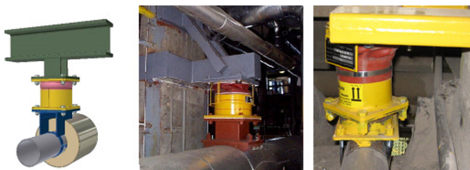
Figure 9. Damper housings attached to the piping and piston attached to the rigid structure.
