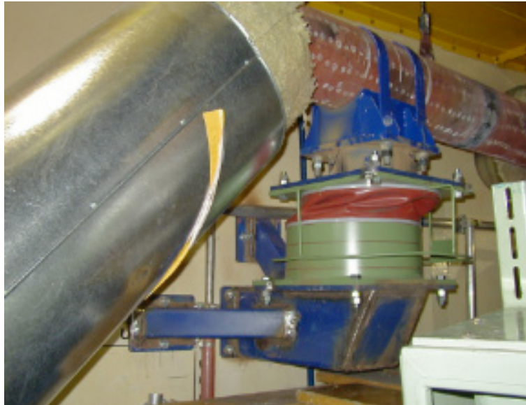
Figure 46. VES damper at the RL76 in RB LO2 during installation. Damper's piston attached to the piping, housing – to the RB wall.
