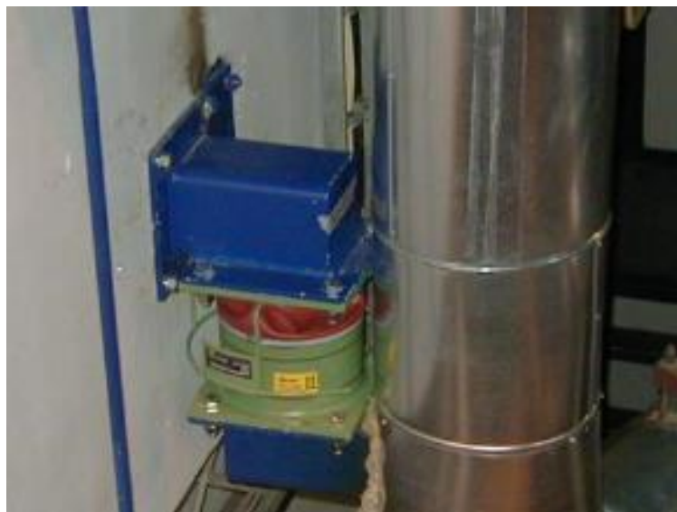
Figure 49. VES damper at RA10 piping in deaerator room. Damper's housing attached to the piping, piston – to the wall.
