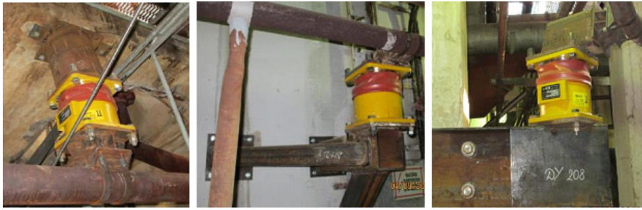
Figure 63. Examples of damper supports installed on interstage piping of compressor No 2.
