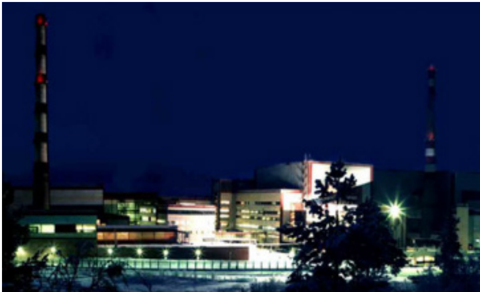
Figure 33. Image of Kola Nuclear Power Plant.
