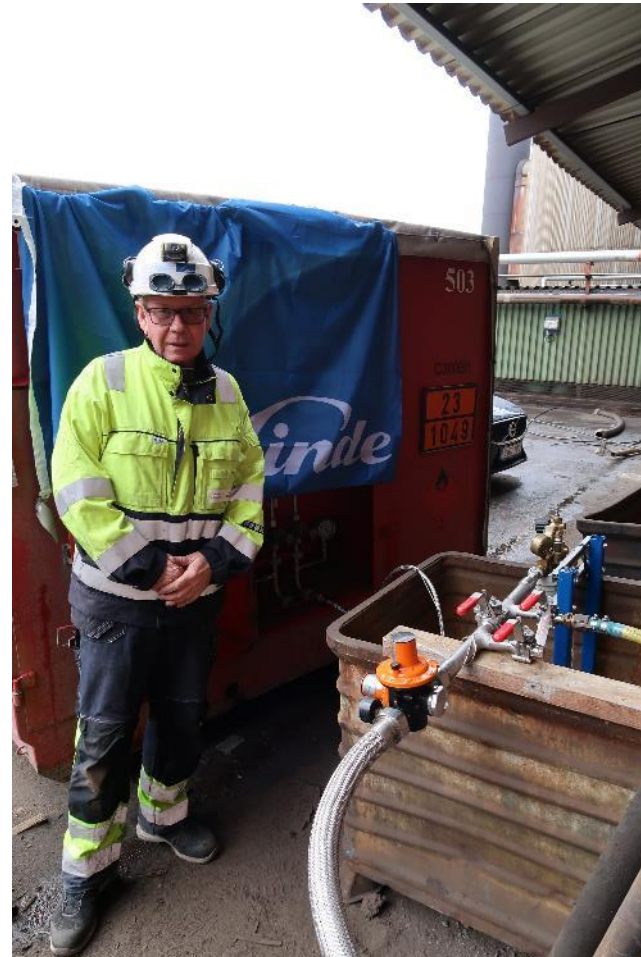
Pressure reducer to 2 bar(g) and slam shut
