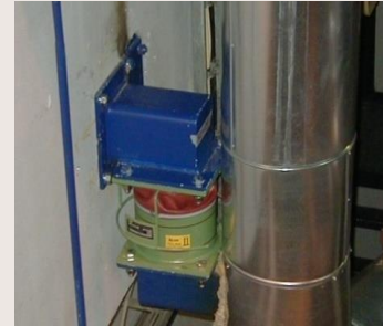
Inverse installation of the VD at the piping
