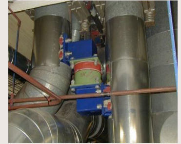
Connection of two piping by VD in the open air using their different dynamic properties
