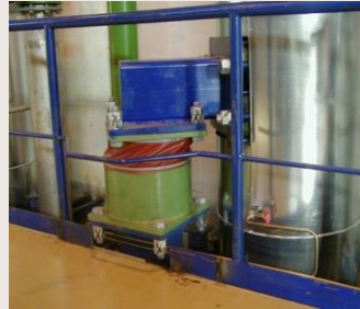
VDs at the main steam vertical run piping
