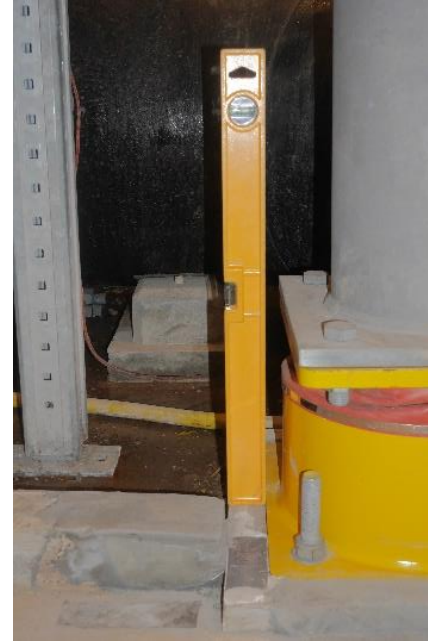
Viscodamper with vertical misalignment to approximately 7-9° (Acceptable 5°)
