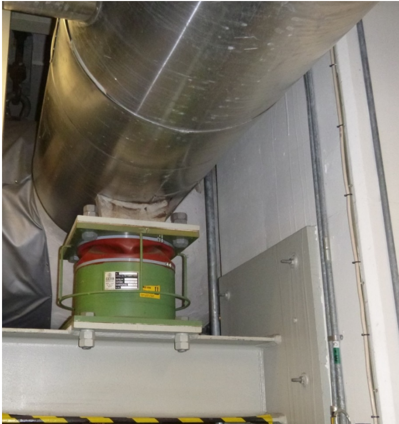
Figure 34: Example of one type of viscous damper and how it is connected to the pipe and supporting steel beam.
