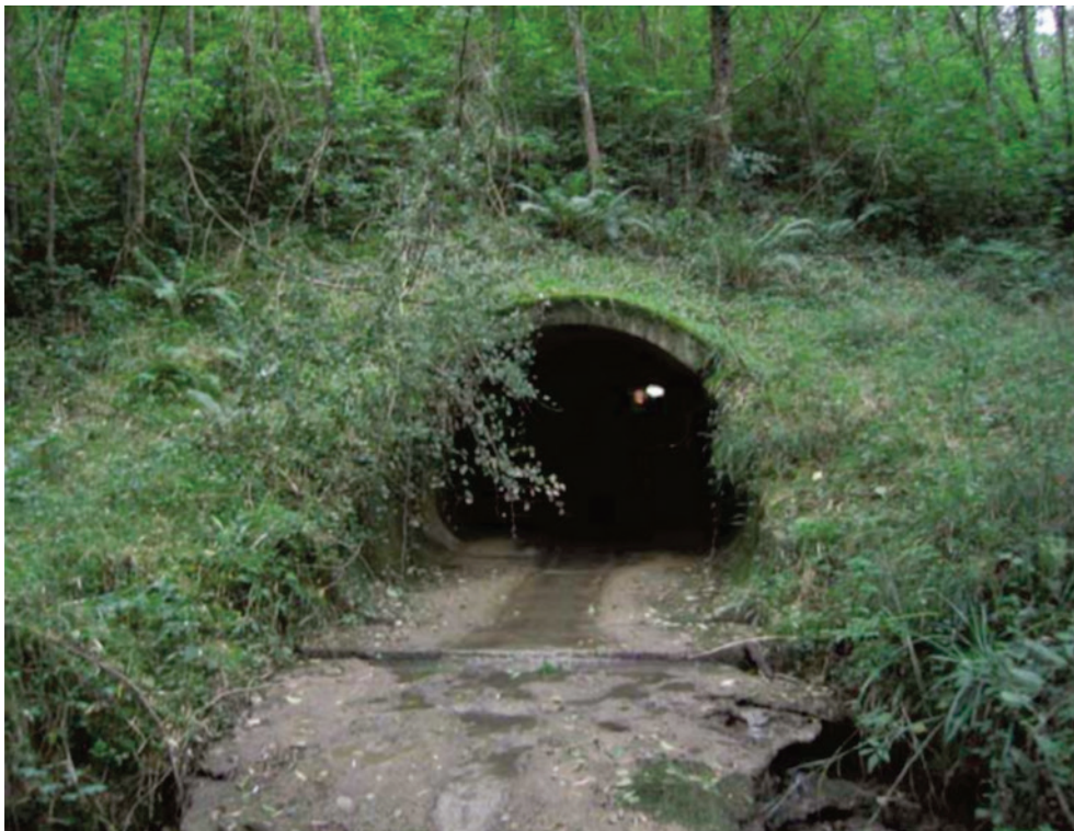
Figure 3. Entrance of the concrete culvert [9].
