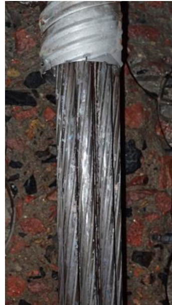
Figure 8 Removal of the duct and uncovering the strands - Waterjetted strands
