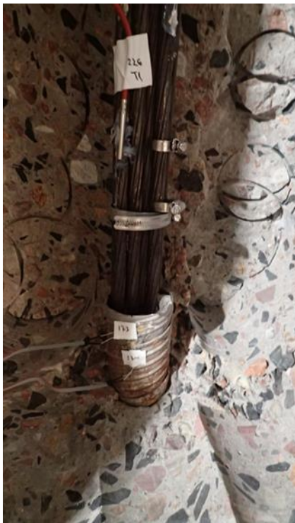
Figure 28 Attachment of strain gauges on the duct, window V5 before and after cutting of the strands
