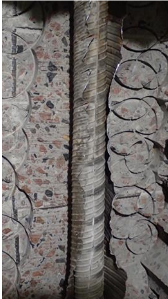
Figure 9 Removal of the duct and uncovering the strands - Cut and unrolled duct
