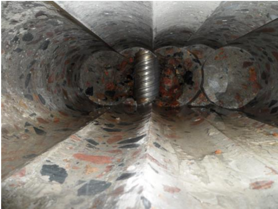
Figure 6 Series of drilling to remove much of concrete within the test window.
