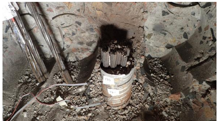
Figure 29 Attachment of strain gauges on the duct, window V5 before and after cutting of the strands
