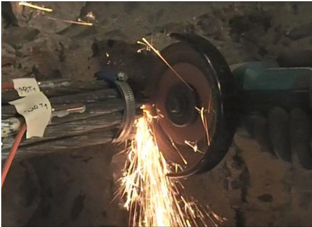
Figure 20 Cutting off the strands by means of an angle grinder.
