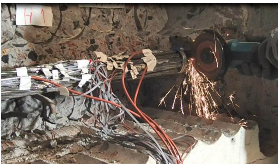
Figure 19 Cutting off the strands by means of a grinder
