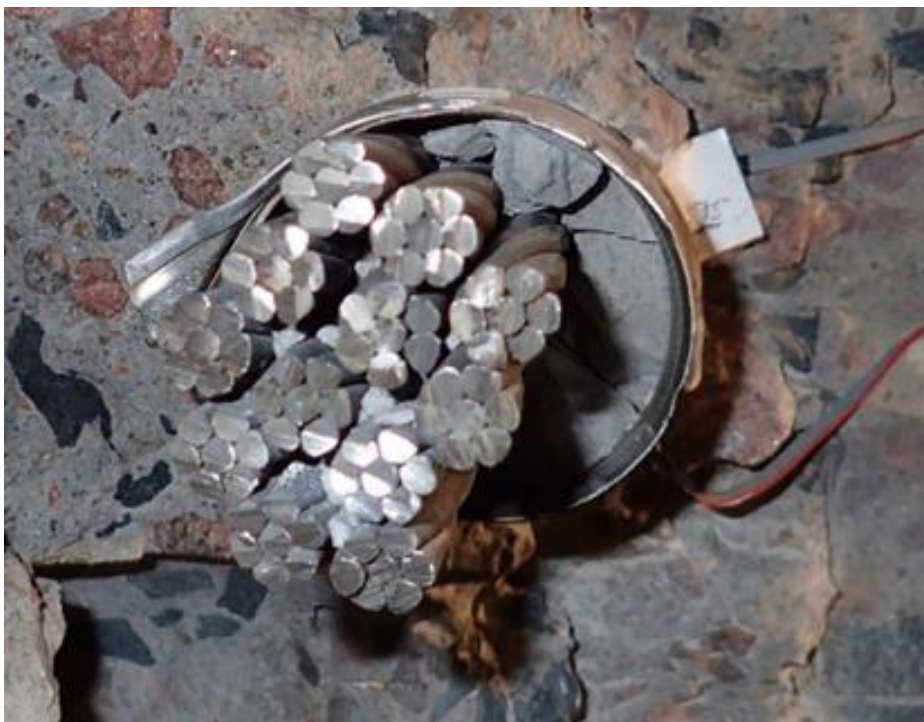
Figure 11 Grout between horizontal strands and duct
