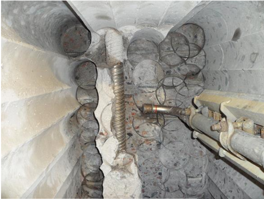
Figure 7 Uncovering the duct by means of an automated waterjetting lance
