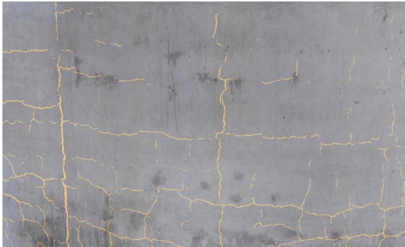
Figure 19. AI-supported high-resolution photogrammetry using drones for remote crack mapping on concrete surfaces. Cracks are highlighted in yellow. Figure from Spotscale.
