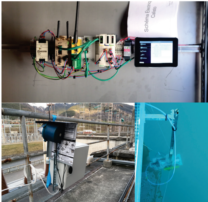
Figur 11. Examples of IoT installations at EDF.
