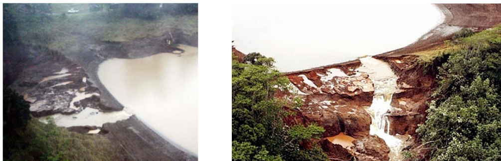
Figur 3-6 Ka Loko Dam – Dammbrott 2006
