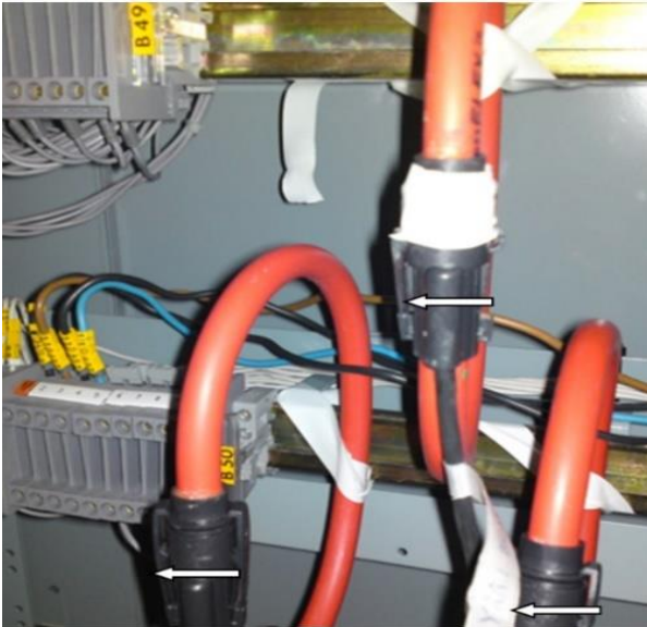
AmpFlex current sensors
