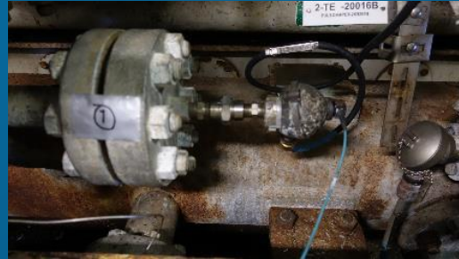
Measurement of thermowell vibration
