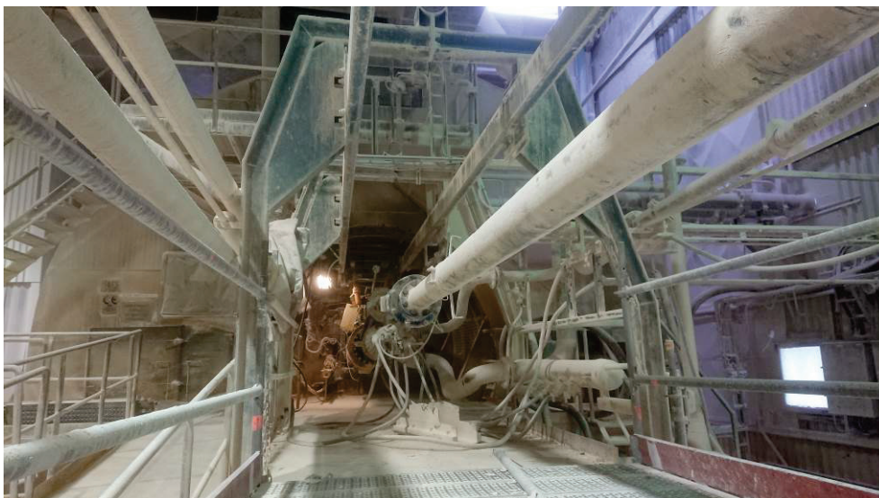
Figure 3. View of the powder burner at one of the lime kilns at the Mönsterås mill.
