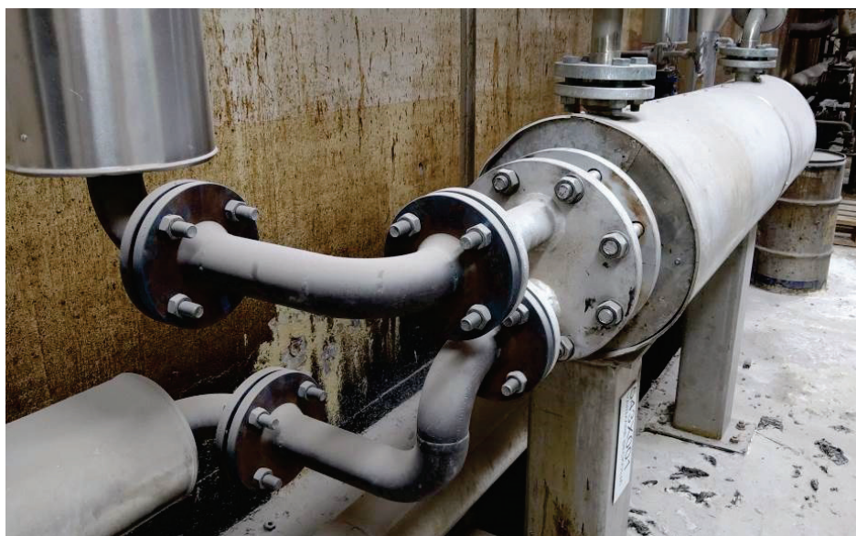
Figure 7. Shell and tube heat exchanger used for preheating tall oil pitch (shell side) in the Gruvön mill. Low pressure steam is used as the heating medium (tube side).
