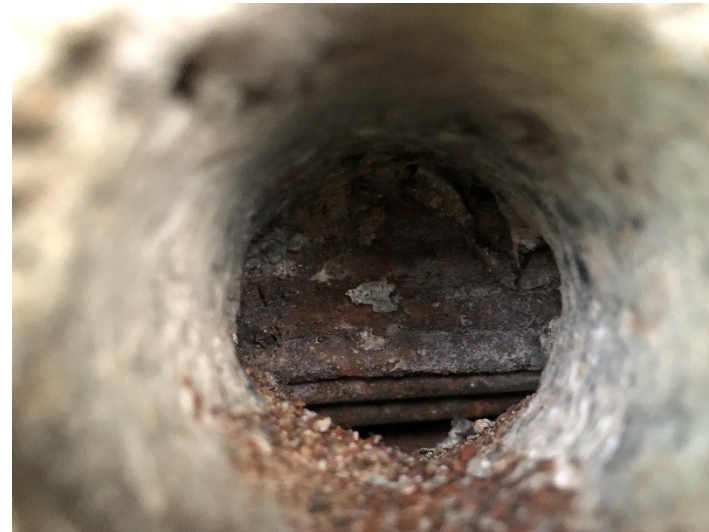
Position of surface reinforcement and prestressed cables
