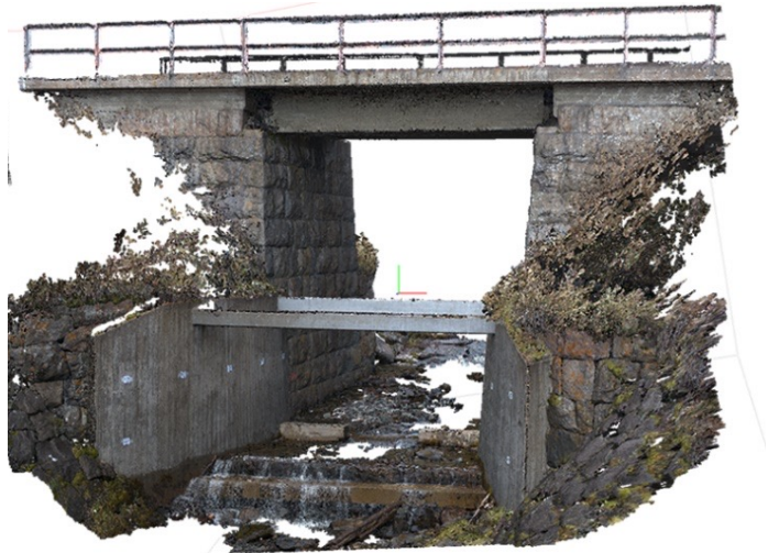
3D model of Juovajokk bridge obtained by photogrammetry
