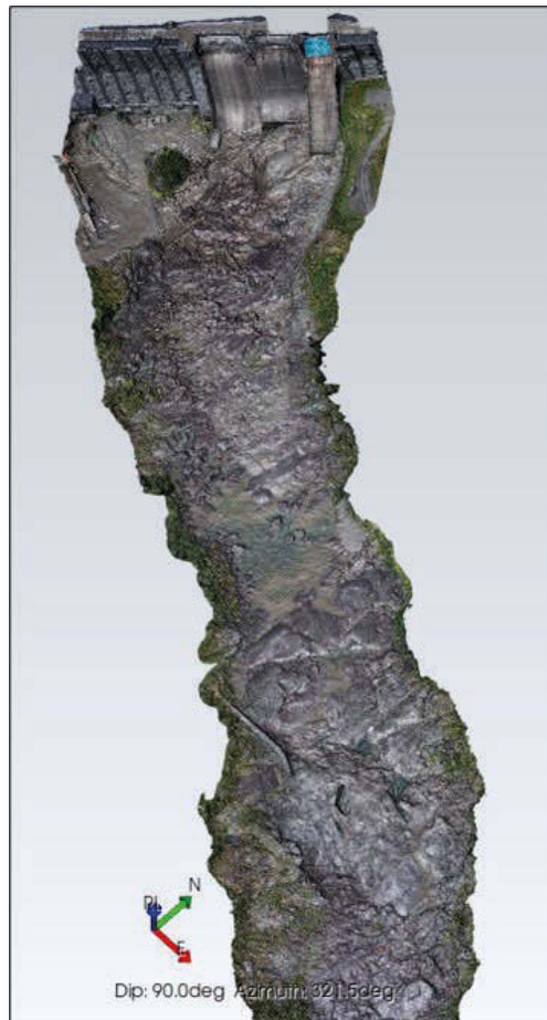
Figure 27. Dam 2 and its spillway channel.
