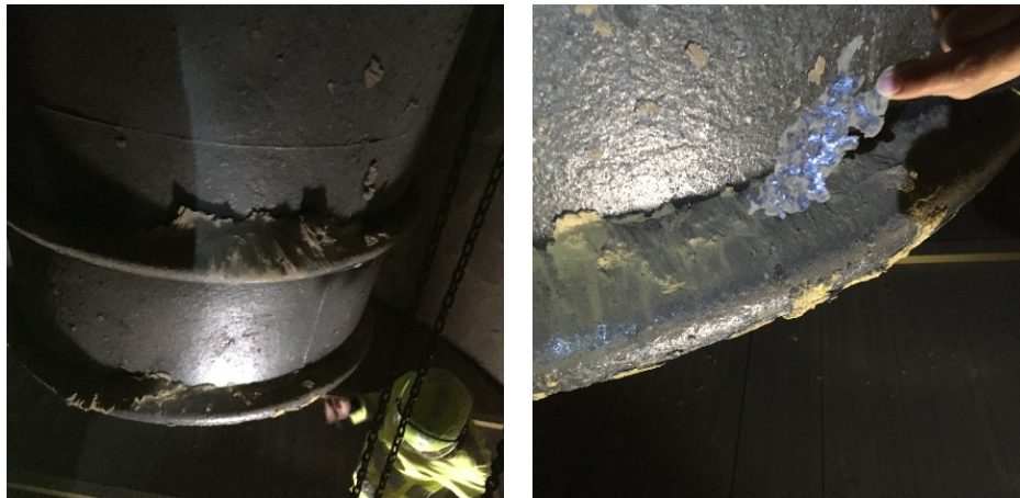
Figure 17 Cyclone vortex finder in Händelö P14 boiler. Flakes from this area were retrieved for SEM/EDS analysis.
