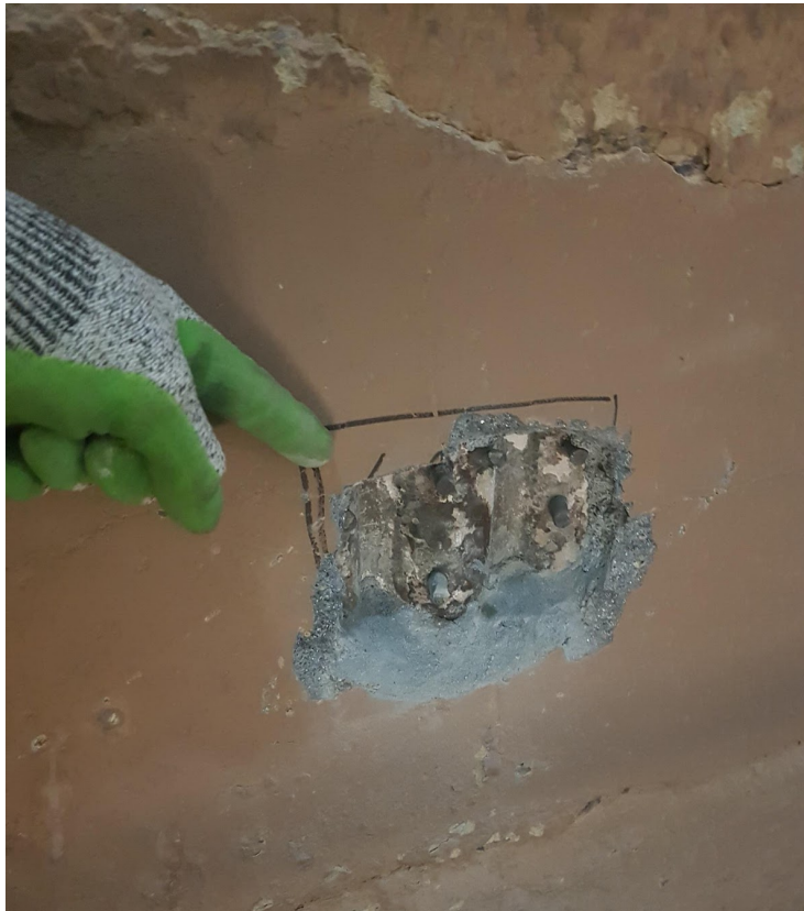
Figure 53 Boiler area after break-out sample was taken, prior to re-casting.
