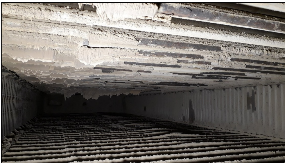
Figure 6 Manhole view at level +5 (evaporator bank) in the boiler Händelö P14. The top row of tubes corresponds to the “roof” position, while the bottom row is the “floor” position.
