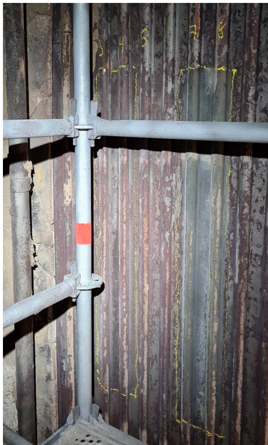
Figure 11. The two areas HVOF sprayed. Tubes 3-4 are metallized with APMT and tubes 7-8 are metallized with CorEr. The image is taken during the first revision, about 1 year of exposure.
