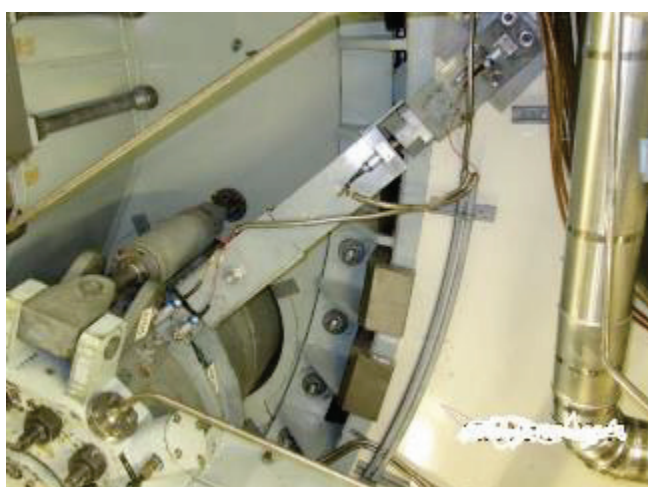
Figure 56: Mitigation enforcement beam installed on MC-pump
