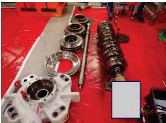
Figure 24: Inspection of pump shafts impeller
