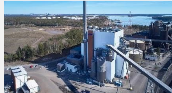
Multifuel to energy
