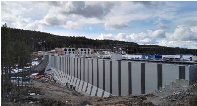
Ramsele buttress dam (Photo: Fortum).
