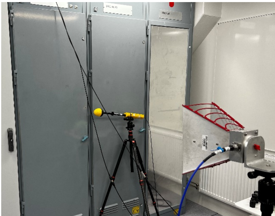
Figure 19 - Testing with the front door of the cabinet closed (Cabinet THE.102)
