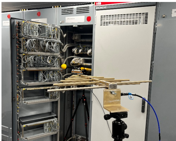
Figure 17 – Testing with the front door and internal panel door open (Cabinet THE.104)
