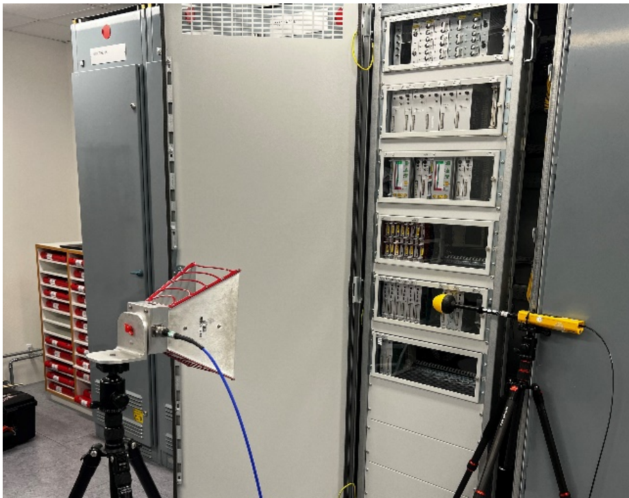
Figure 18 - Testing with the internal panel door closed (Cabinet THE.103)
