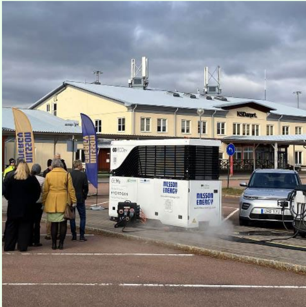
Electricity to go – fuel cell generator
