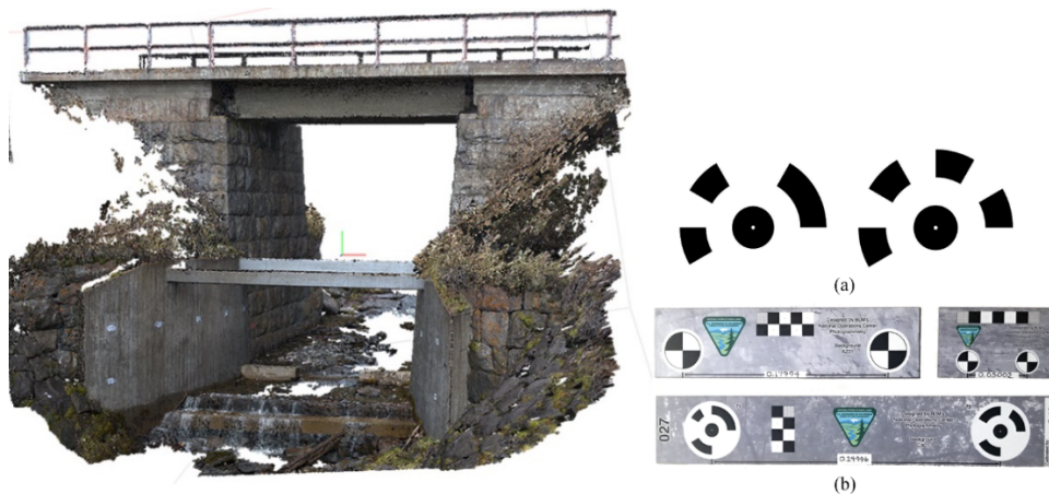
Figure 3-19. Left) Ground-based photogrammetry camera for Juvajokk Bridge; Right) Artificial targets used in the alignment process and for scaling: (a) coded targets and (b) calibration scale bars.
