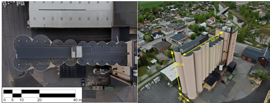
Figure 4-4 Dimensions of the inspected concrete silo.
