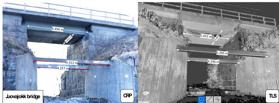
Figure 3-20 Measurements of bridge structural elements in both CRP (left), and laser scanning (right) method.
