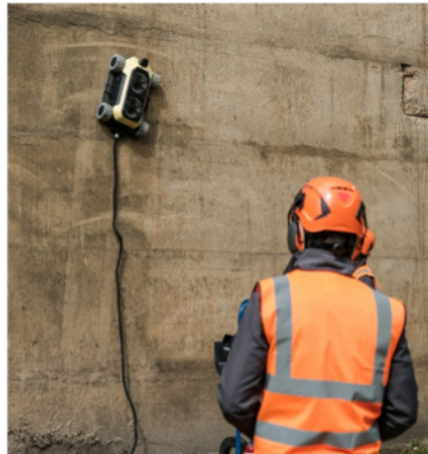
Automated wall-climbing robot, designed by Hausbots ( https://hausbots.com/ )
