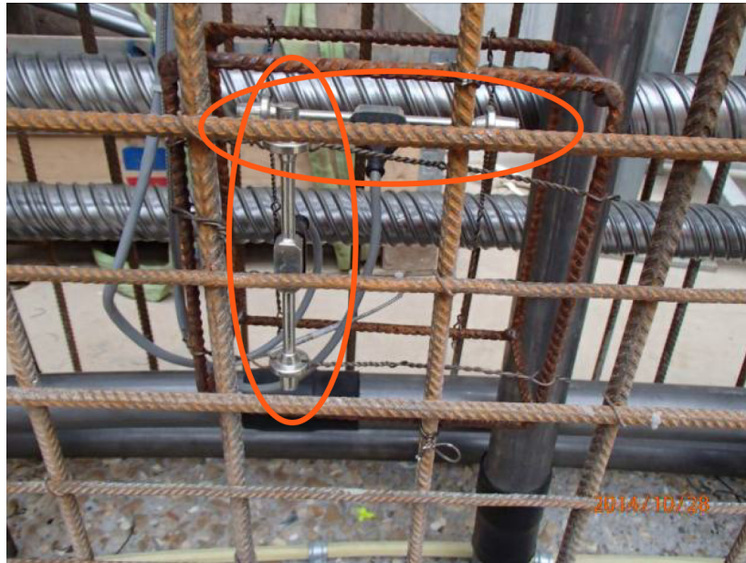
Figure 4—9 Two strain gauges mounted in a rebar cage before casting. Oukhemanou, (2016).
