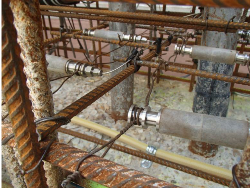
Figure 6—7 Pulse sensors to be cast into concrete, Oukhemanou (2016).
