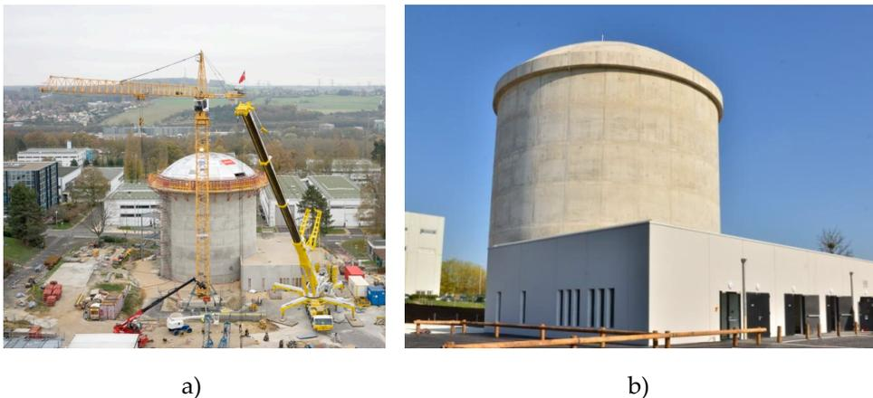
**Figure 1.1 Photo of the construction of the VERCORS mock-up in scale 1/3., from [1]**
